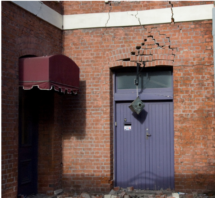
Figure 21. The form of the arches over the doors on the west elevation (left) and the lean-to (right).
