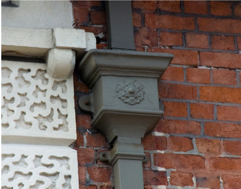
Figure 30. The downpipe on the west elevation.
