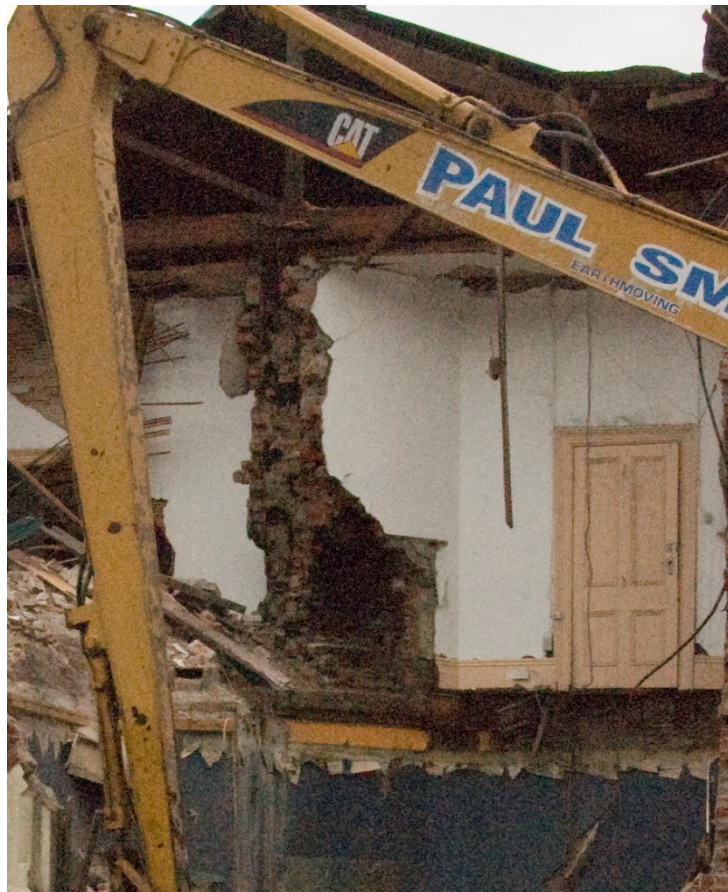
Figure 41. The first floor corner fireplace.
