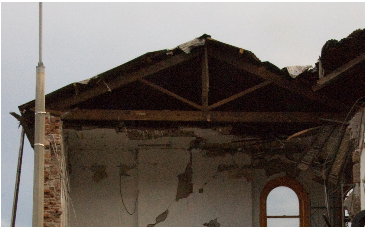
Figure 12. The roof trusses in the east bay of 7 Norwich Quay.
