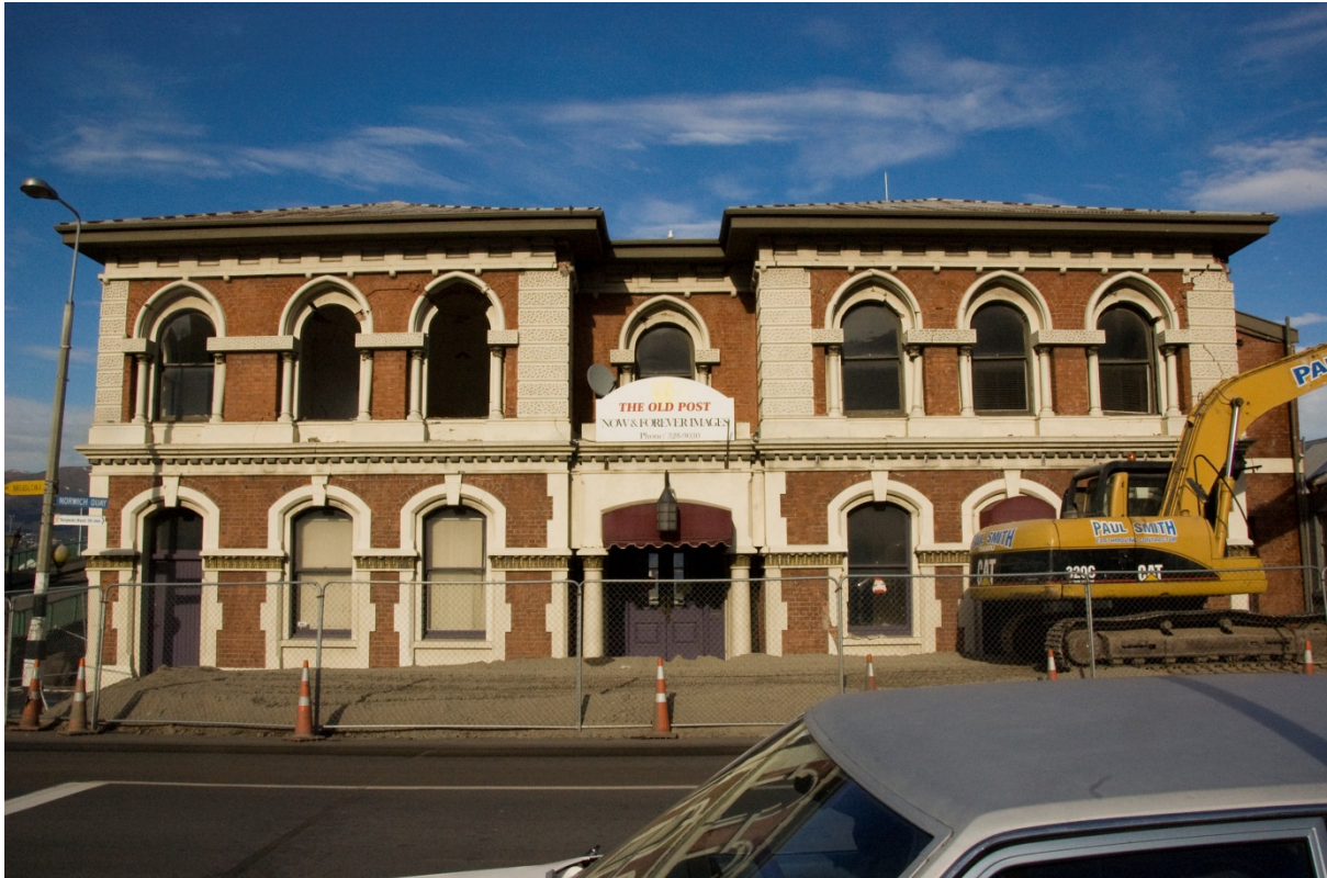
Figure 23. The north elevation of 7 Norwich Quay.
