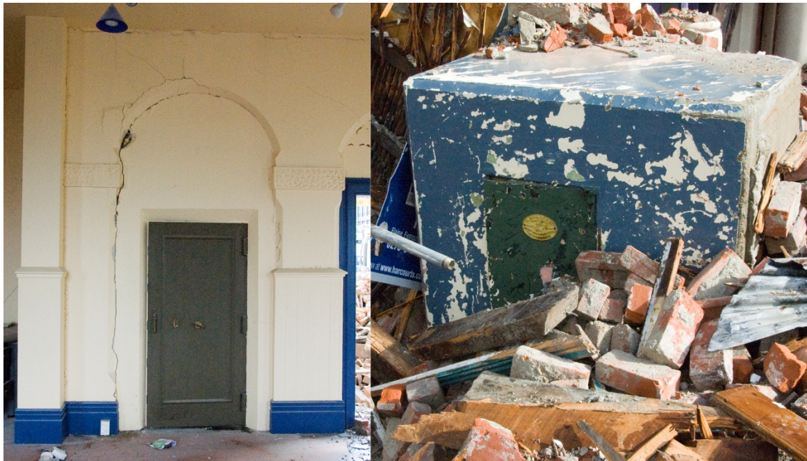
Figure 35. Left: The door into the safe. Note also the timber dado and the vermiculated quoins on either side of the door. Right: The safe.
