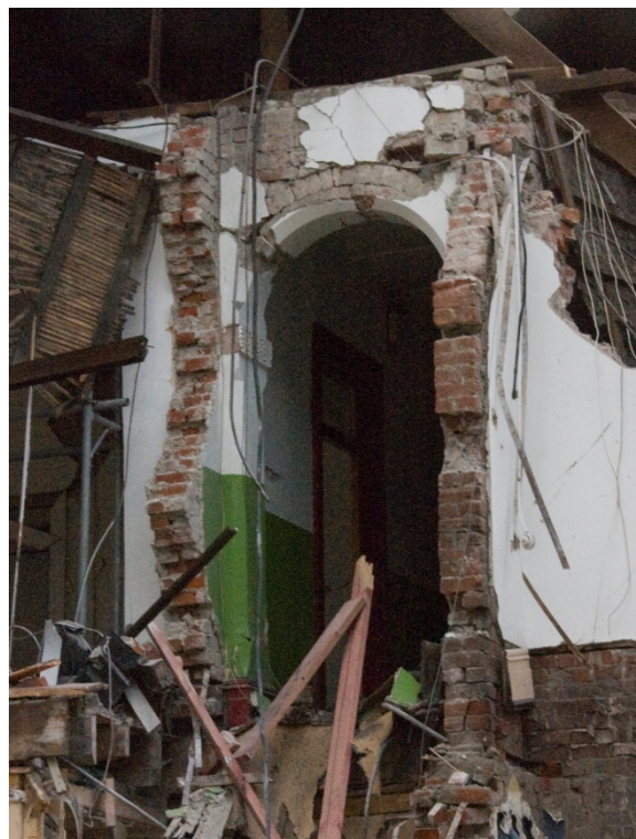
Figure 43. An arched door in the first floor hallway.
