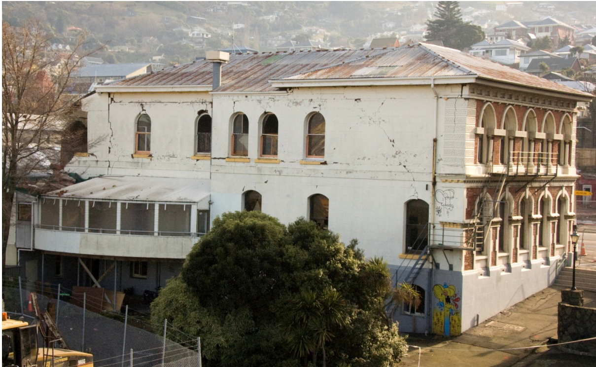
Figure 28. The south elevation.
