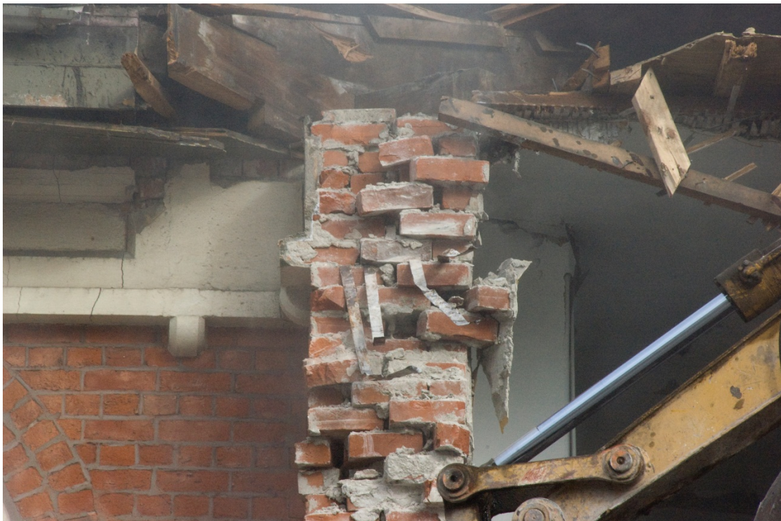
Figure 6. The brick walls of the first floor of 7 Norwich Quay, showing the English bond brickwork and the hoop iron used as reinforcing. Note, however, that in the 16 courses of brickwork shown, there is only one layer of hoop iron reinforcing.
