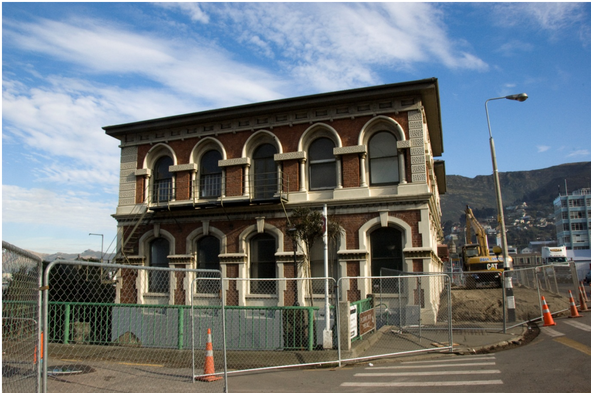
Figure 27. The east elevation.
