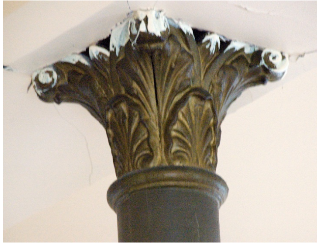
Figure 37. The capital of one of the metal columns in the restaurant.
