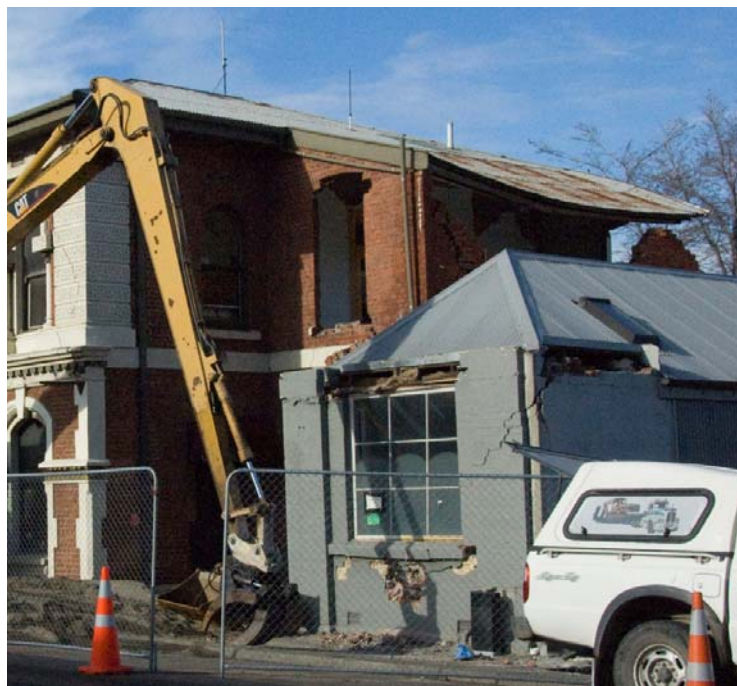
Figure 29. The west elevation.
