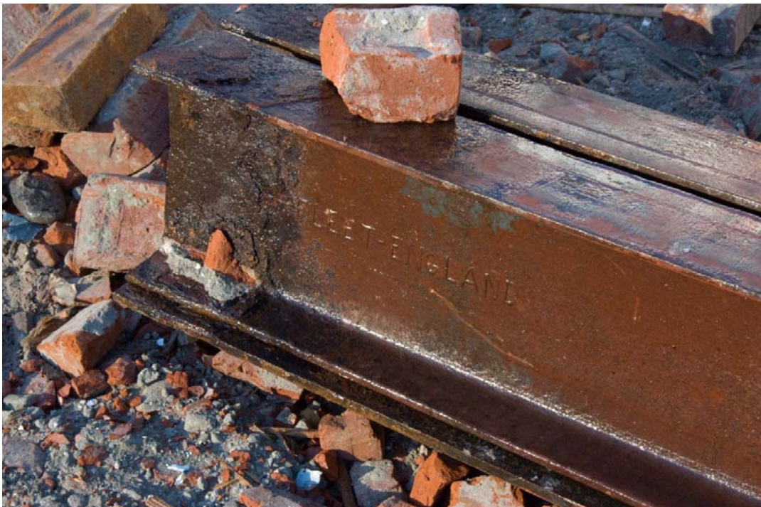
Figure 16. Two Cargo Fleet I-beams that were bolted to a metal plate.
