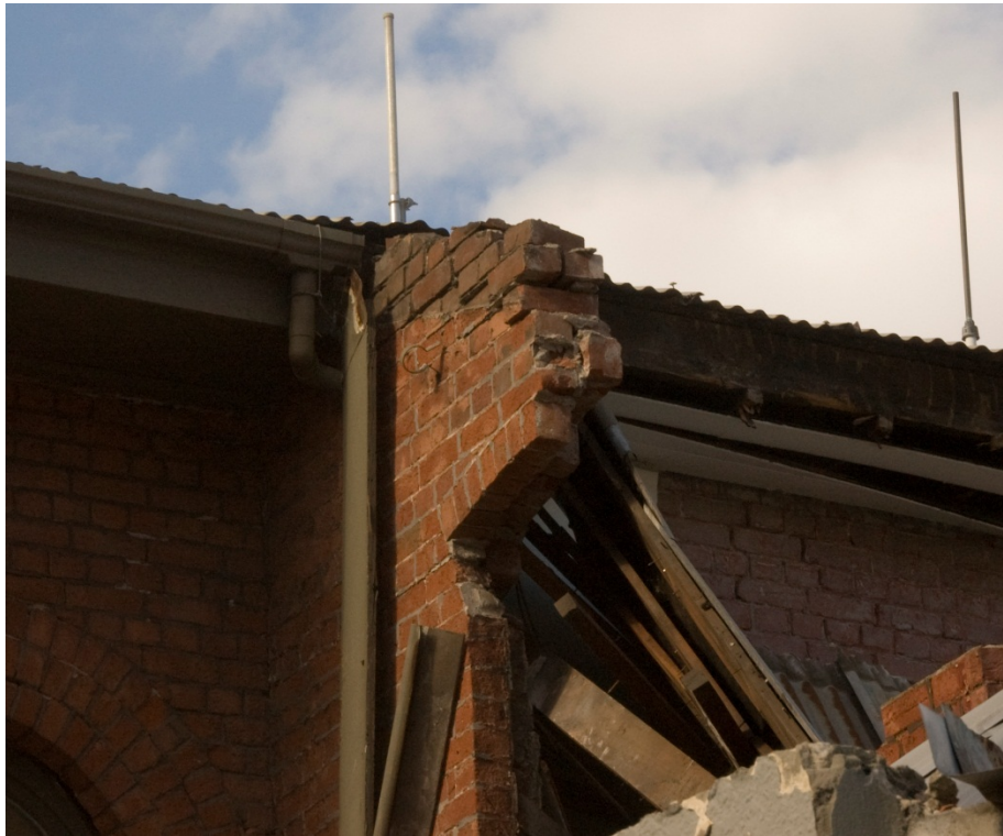
Figure 10. The north wall of the lean-to, showing the brickwork.
