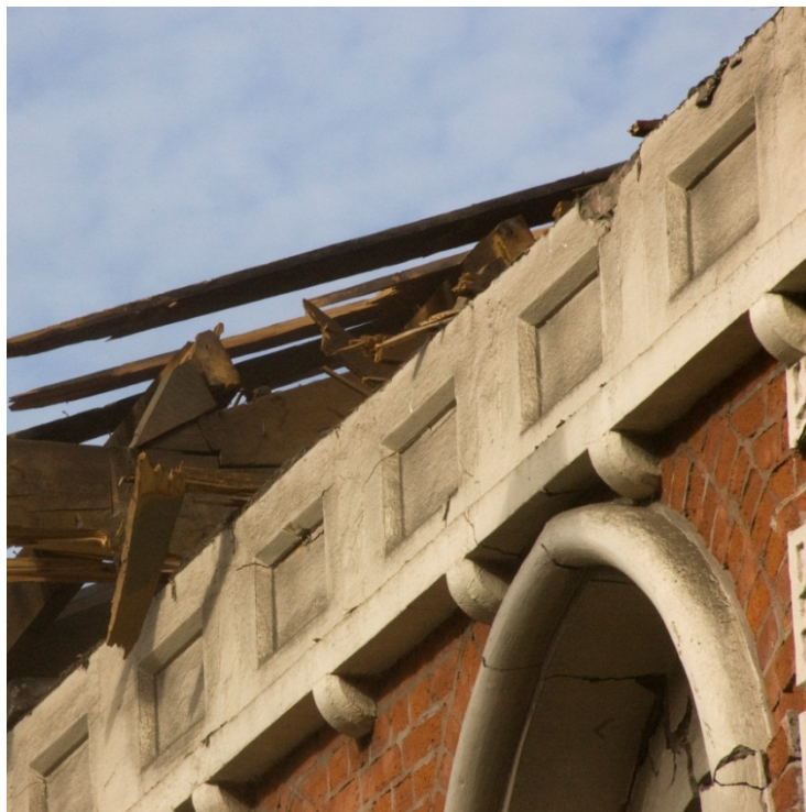
Figure 26. The string course immediately below the eaves of the building.
